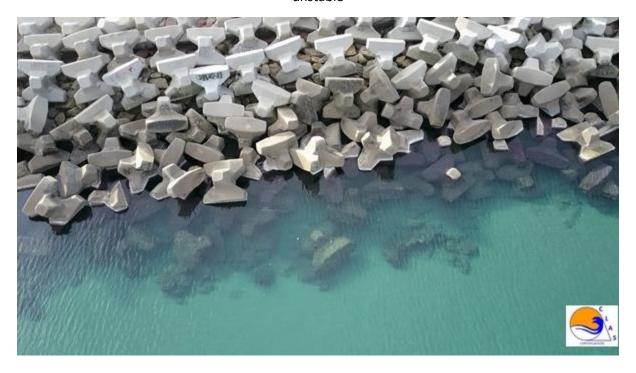
ACCROPODE<sup>™</sup>, ACCROPODE<sup>™</sup>II, ECOPODE<sup>™</sup>, CORELOC<sup>™</sup> and X-bloc<sup>®</sup> CLASS C armours need to be rebuilt.
