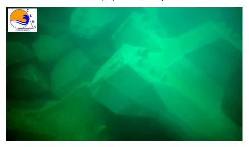
Block totally out of profile not detected by the tools of installation and inspection on DAS ISLAND. This pose was approved based on ECHOSCOPE survey witch not allows to see out of profiles. We supervised as a third part the repair of 5000 meters of X-bloc® shell.
