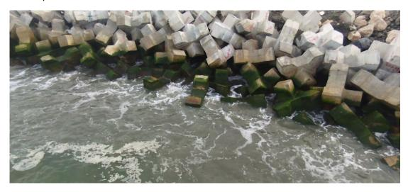
The presence of these bubbles in the water disturbs the image that no longer allows to lay the blocks.
