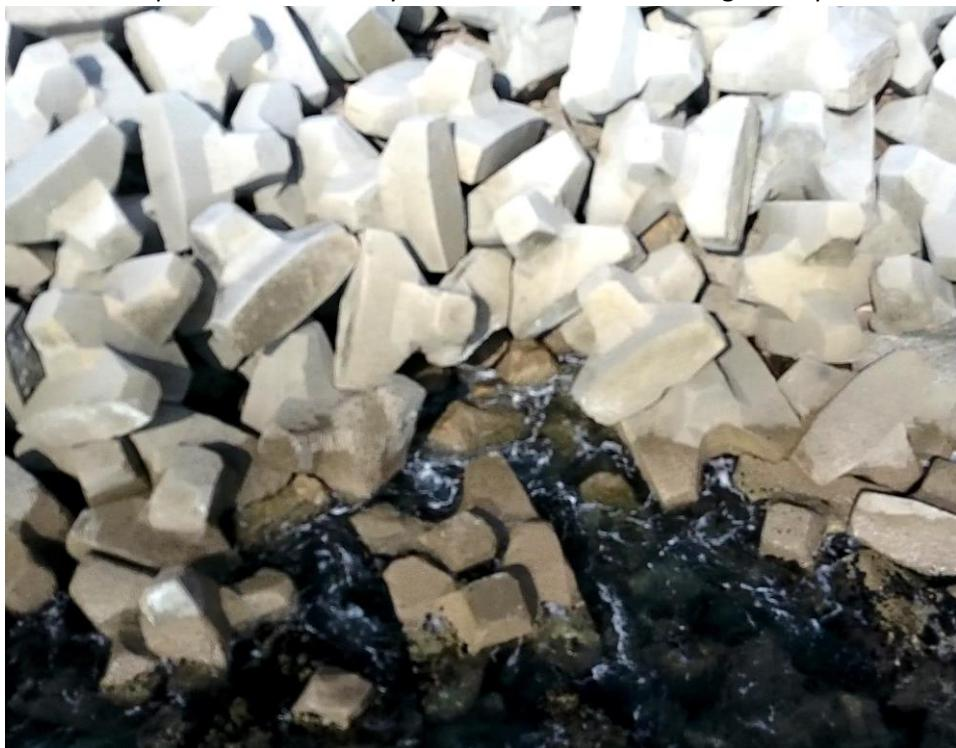
Contact faults always exist after construction, even when you do not leave any. But when they are rare, it does not matter. This is why during construction CLAS inspectors report and repair missed contact. So the problem remains too marginal after the construction to cause disorders.
