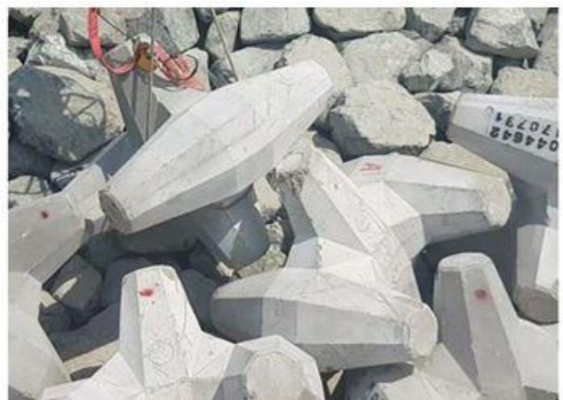
The strength of the carapace and its durability strongly depend on the quality of the interlocking. CLAS has used and tested all commercially available inspection and construction assistance tools including ECHOSCOPE®, POSIBLOC™ and DIDSON and ARIS acoustic cameras. Until now only a specially teached and trained human can avoid the accumulation of harmful contact defects in ACCROPODE™, ACCROPODE™ II, CORELOC™, ECOPODE™ and X-bloc® construction.
