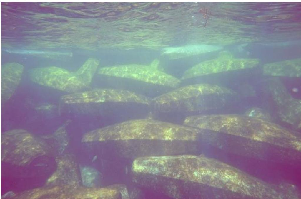
Block broken due to a movement due to a contact fault
