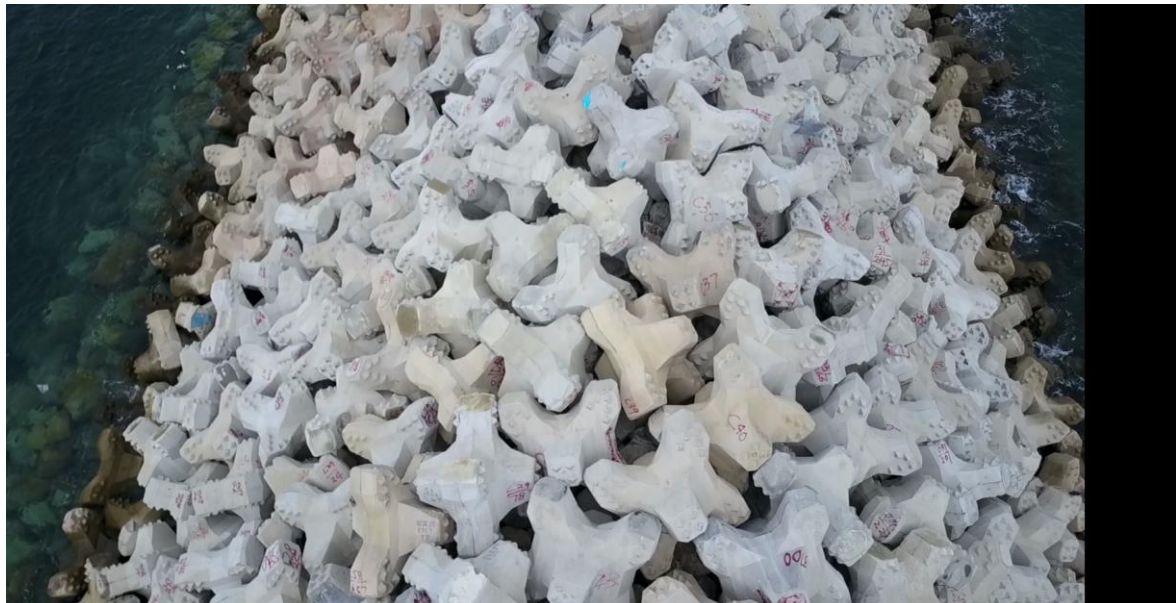
Drone inspection of an ACCROPODE™ II armour crest
