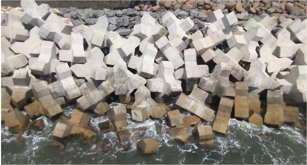
X-bloc® inspected by drone
