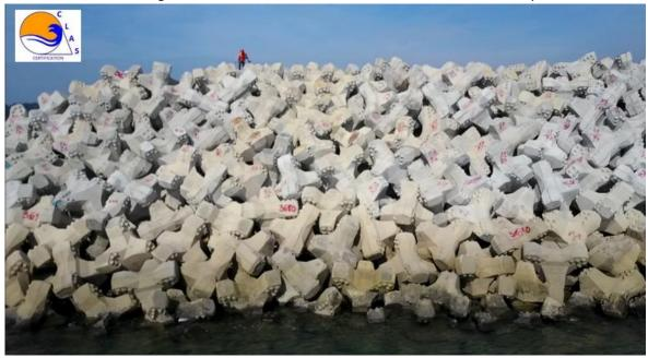
Based on the reports of TECHNOLOGY COMPLIANCE prepared by the CLAS inspectors, the ACCROPODE<sup>TM</sup>, ACCROPODE<sup>TM</sup>II, ECOPODE<sup>TM</sup>, CORELOC<sup>TM</sup> and X-bloc<sup>®</sup> armour can be unreservedly approved as conforming to the design and technology and validated CLASS A armour construction.
