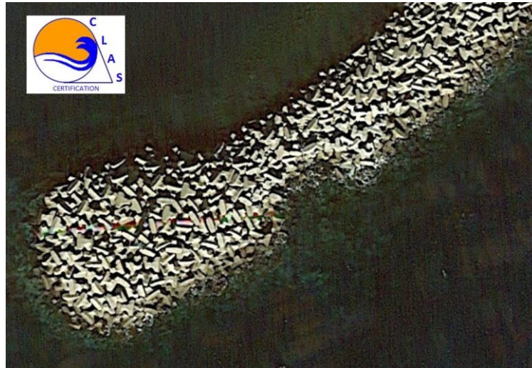
ACCROPODE™ armour partly destroyed
